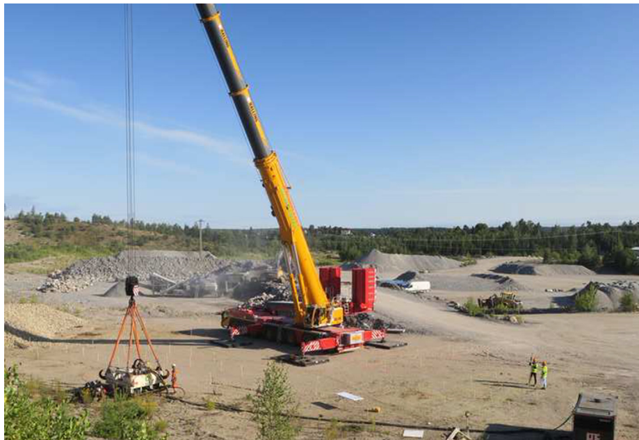
Fig. 1. Test site with compactor (left), power pack (right) and lifting crane.
