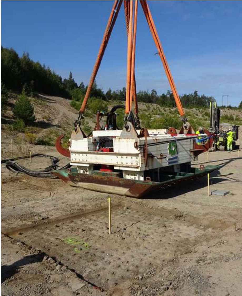
Fig. 6. The HVP compactor (background) and settlement imprint resulting from compaction (foreground).
