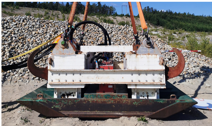
Figure 1: Photo of the HVP-compactor at the Älvnäs site.
